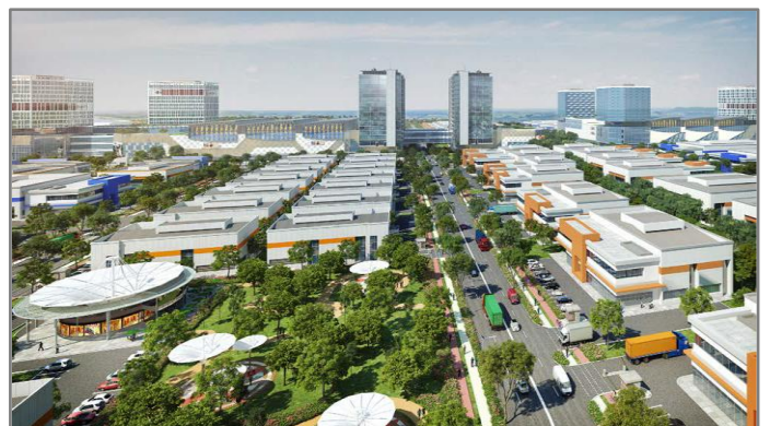
BEST INFRASTRUCTURE PROJECT 2019 | SIP MEMBERS | SILVER AWARD VISAKHAPATNAM-CHENNAI INDUSTRIAL CORRIDOR (VIC) Andhra Pradesh, India Surbana Jurong Consultants Pte Ltd
