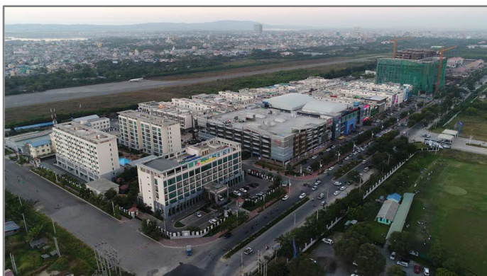
BEST INFRASTRUCTURE PLANNING PROJECT 2017 | SIP MEMBERS | MERIT AWARD INFRASTRUCTURE PLAN FOR MINGALAR COMMERCIAL PLAZA Mandalay City, Myanmar SCP Consultants Pte Ltd
