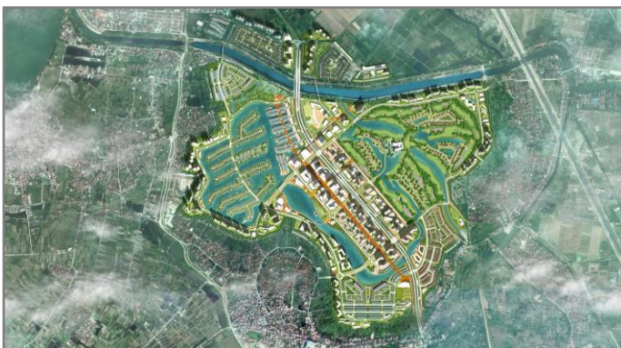
BEST PLANNING PROJECT 2017 | SIP MEMBERS | SILVER AWARD ECOPARK 2016 MASTER PLAN REVISION Hanoi, Vietnam CPG Consultants Pte Ltd
